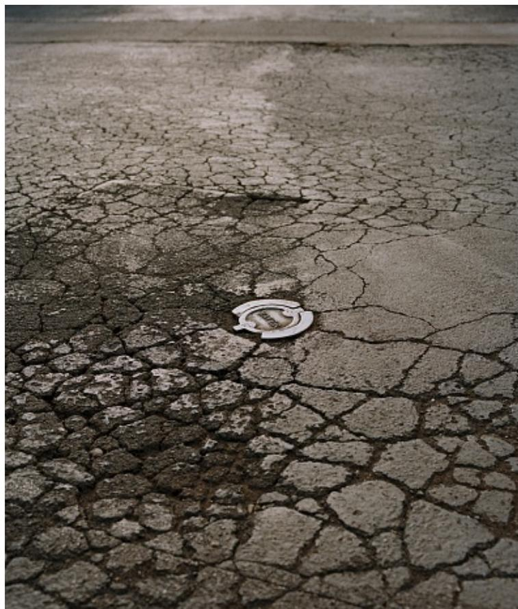
Cracked asphalt on the roads at Shadowbrook
